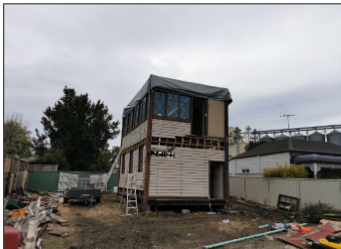
The signal box has been tidied up and stripped back ready for transportation to Harcourt. The stairs and verandah will be transported separately.
