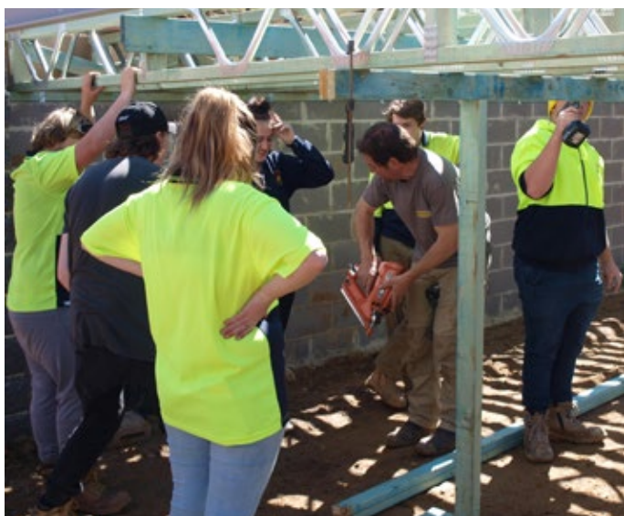
Tim Meir, supervisor, demonstrates the use of a staple gun. Here the students are working on the underfloor of the station building. The space they are working in will be used to store engines and carriages. The platform will be constructed above and to the left of the storage space.
