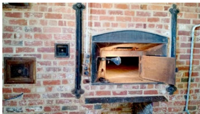
The oven with the new floor; note the electronic sensor wires coming out of the wall in the bottom left hand corner. This modern addition has been made approximately 98 years after the oven was constructed.
