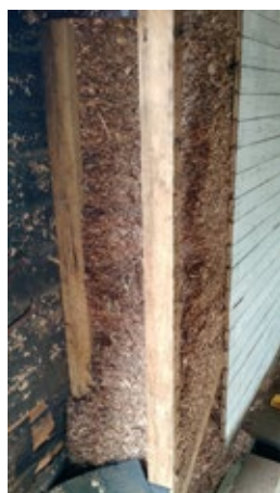
Tightly packed wood shavings fill the walls of the Coolstore.
