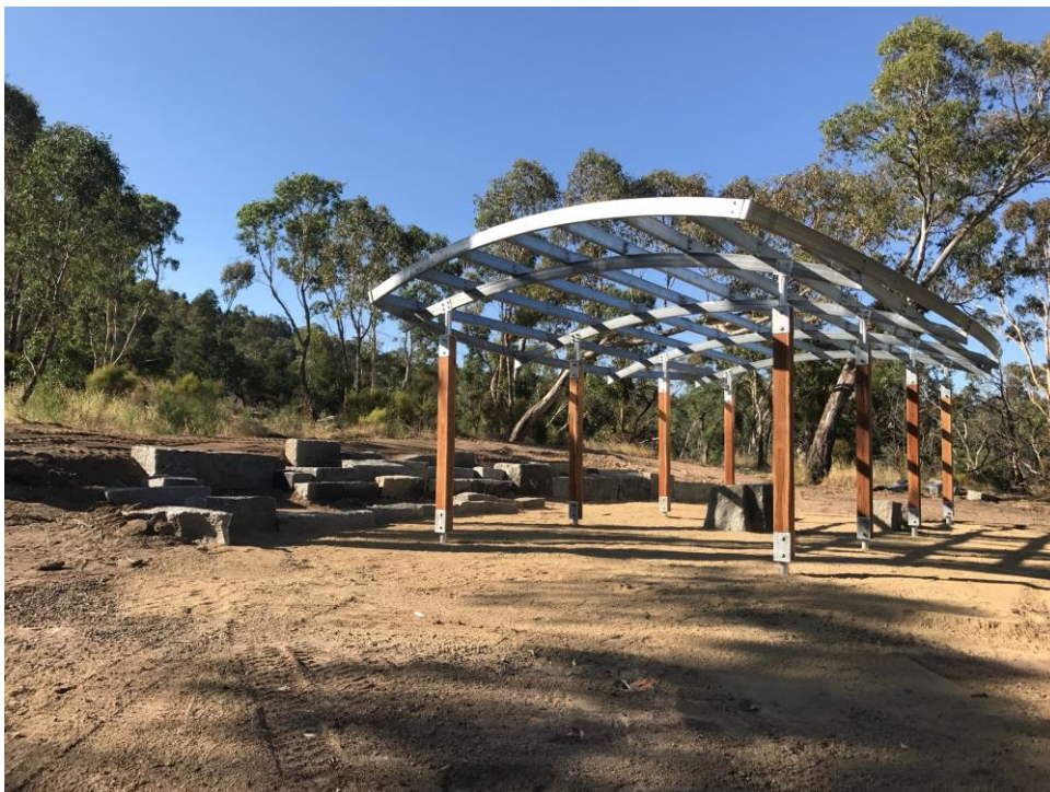
Above: Shelter under construction at La Larr Ba Gauwa Park
